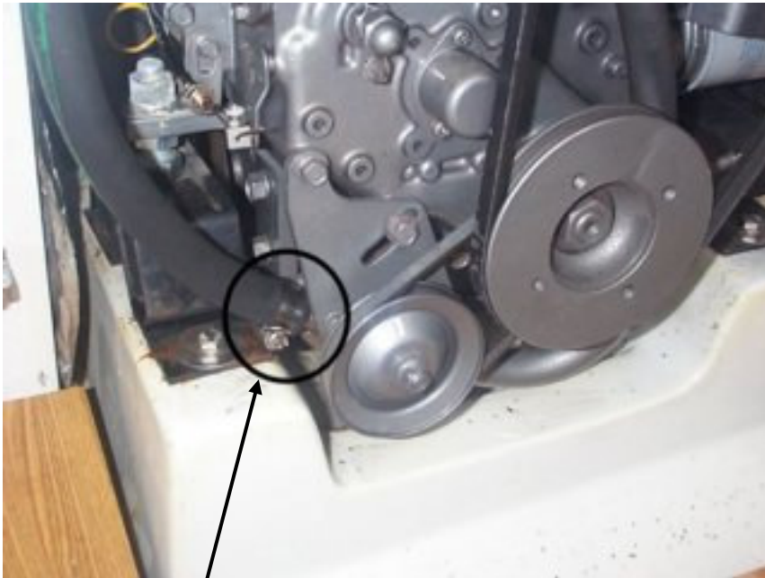
Location of hose that came off engine
